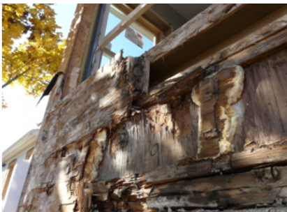
Damage of sheathing and structural components due to water intrusion
