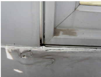
Damage of sheathing and structural components due to water intrusion
