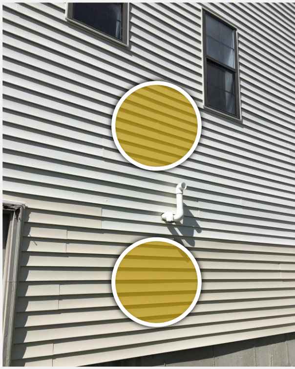
Previous repair performed, Note: different shades of vinyl siding.
