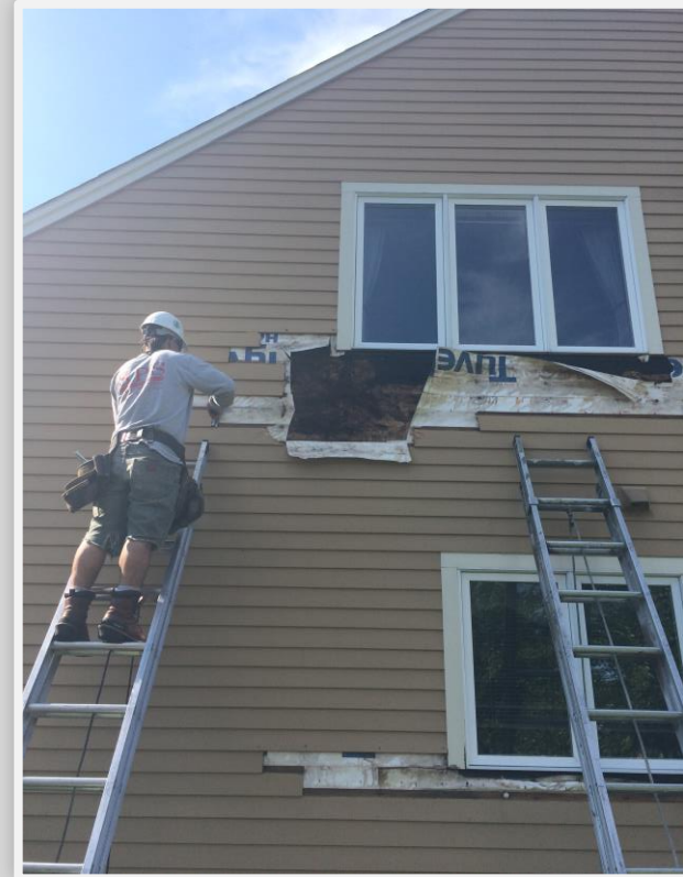
Verified envelope failure
